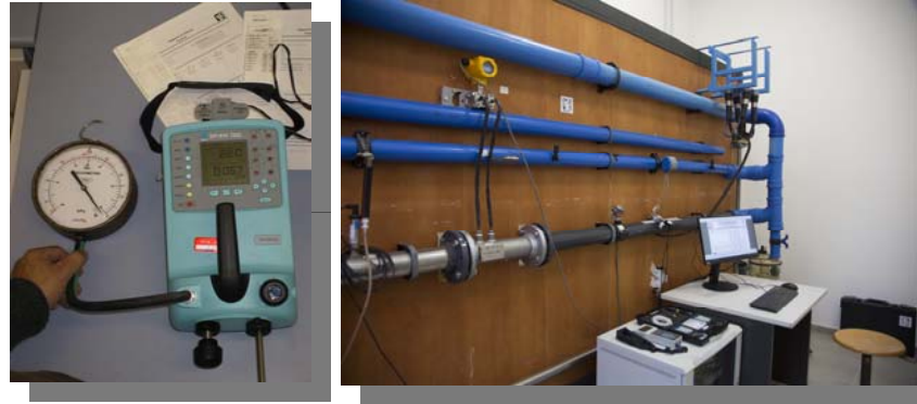
Metrological lab - AIA
